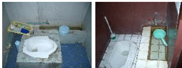
Photo 9 Toilet and water storage tank
